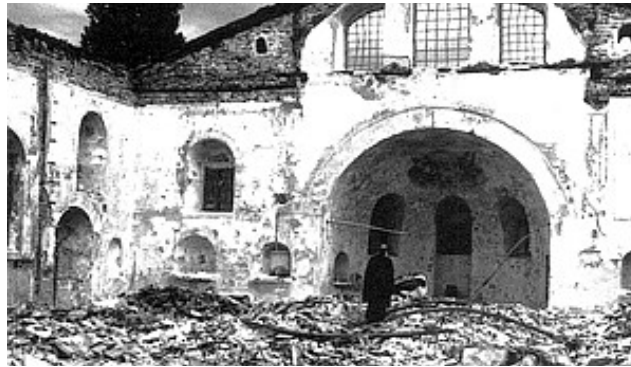
Patriarch Athenagoras prays before the overturned altar table of the destroyed Panaghia Church in Belgratkapi
